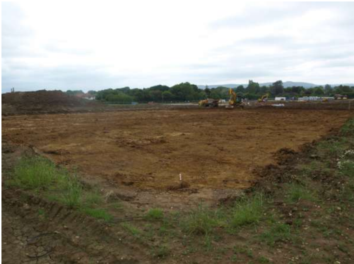
Plate 18: Showing exposed Area 5. Looking south-west.
